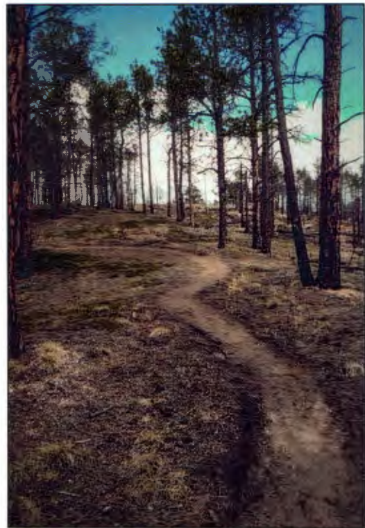
Figure 30 - Typical Hand-Built 18"-24" Singletrack Trail. This Section is Located in Pineries Open Space.
